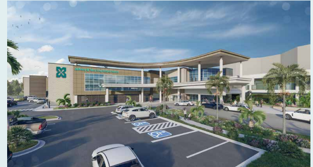
Groundbreaking for Johnny and Terry Gray Surgical Institute Opening 2023
